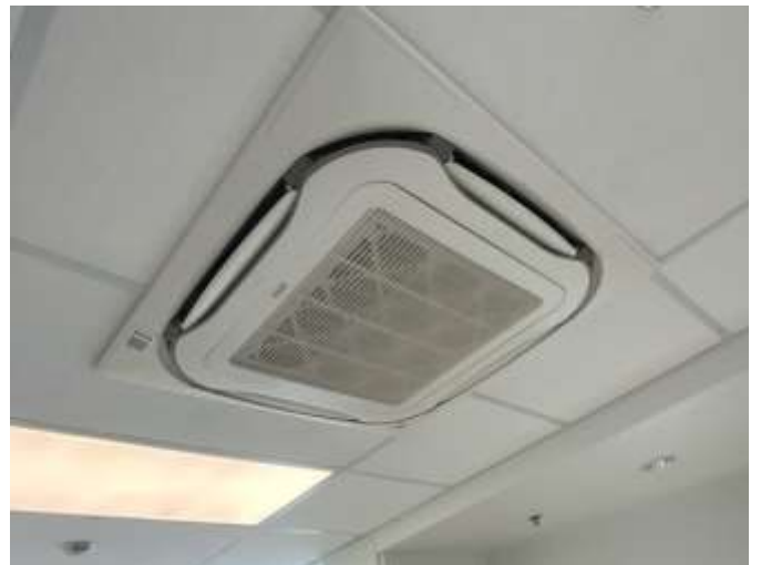
16 - TYPICAL FAN COIL CASSETTE
