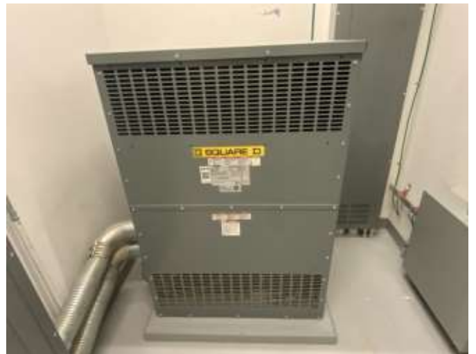
22 - SECONDARY TRANSFORMER
