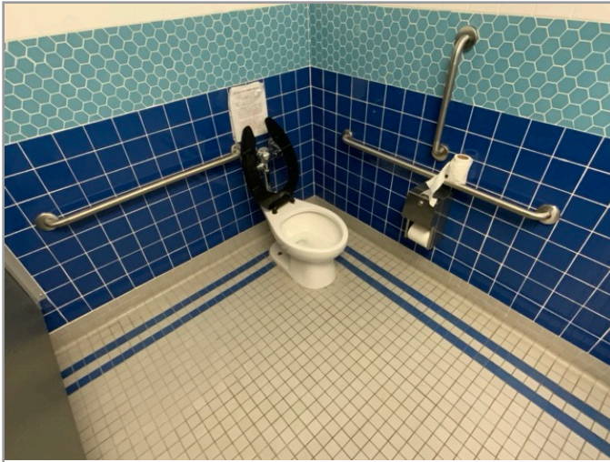
TOILET STALL OVERVIEW
