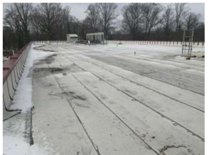
6 - MODIFIED BITUMEN ROOFING
